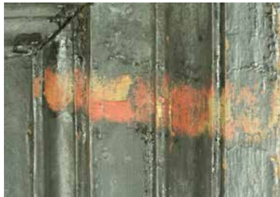
Fig. 22 Detail of fig. 8: polychromy of center frame. Photo: Caroline van der Elst
